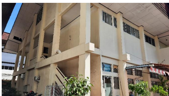
Gambar 6. Tampak Belakang Gedung Graha Bhakti Praja
